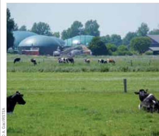
A methanation plant in Germany.
